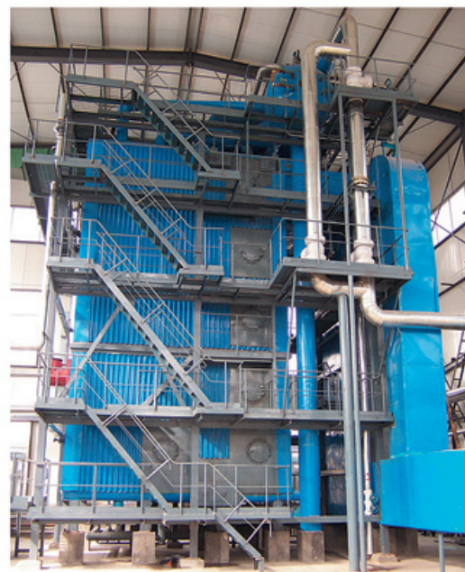
蒸汽锅炉 1×40t/h 煤焦油/重油/干气 中国石油大学 中国2004 Steam boiler 1×40t/h Coal tar/Heavy oil/Gas China oil university China2004
