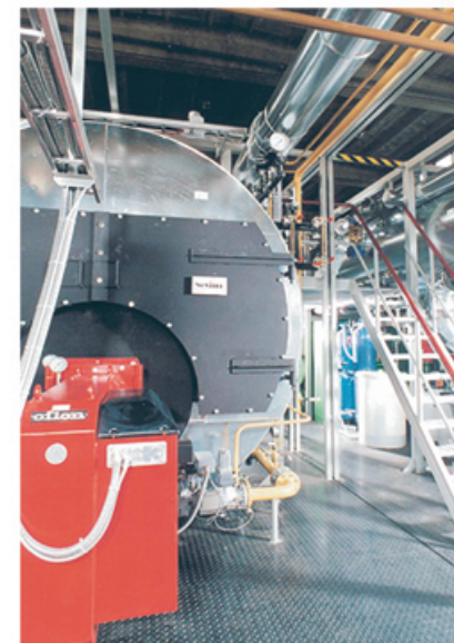
厂制模块化蒸汽锅炉站 15.4t/h 天然气/轻油 Lzhevsk 俄罗斯1999 Modularize steam boiler plant 15.4t/h Natural gas/light oil Lzhevsk Russia 1999
