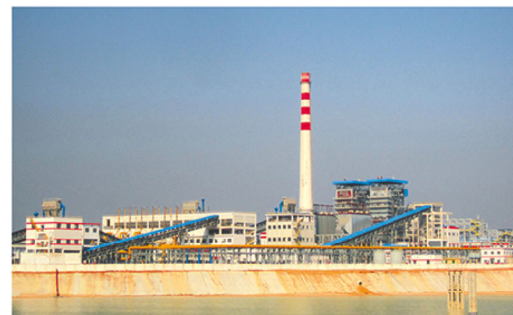
出口越南循环流化床锅炉现场 (TG-170/5.3-M) CFB Boiler Exporting to Vietnam (TG170/5.3-M CFB)
