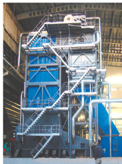
OXL70MW 热水锅炉 70MW Hot Water Boiler
